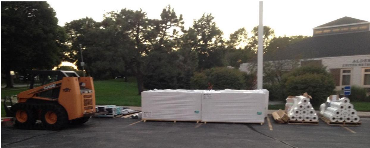
**Roof Insulation.** The stack of insulation in the middle of the picture, above, provided an additional 1” of insulation on the roof. This was a 25% increase.
